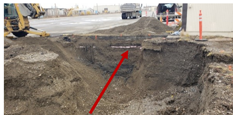
Location of Contamination
