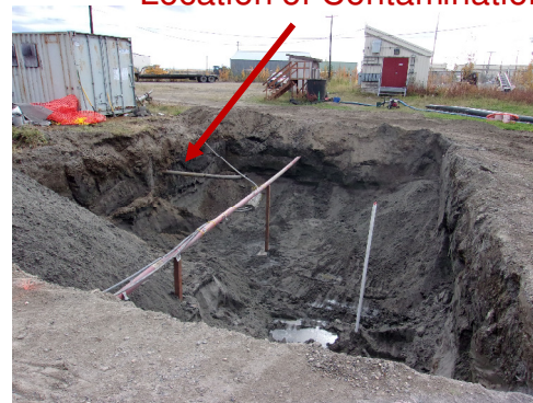
2019 Site SS018 Excavation
